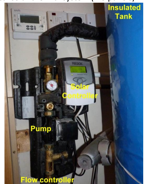
The System at Penybanc B&B Drefach Felindre heating 2 water tanks in adjoining houses - a total of 5 bathrooms
