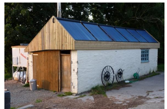
The 15kW system at Ceridwen in Drefach Felindre
